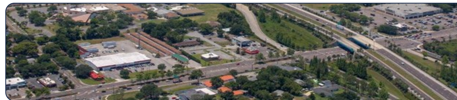
Polk Parkway and South Florida Avenue
